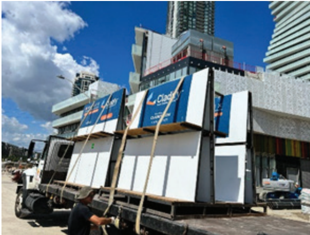
Figure 4: Transportation to site
