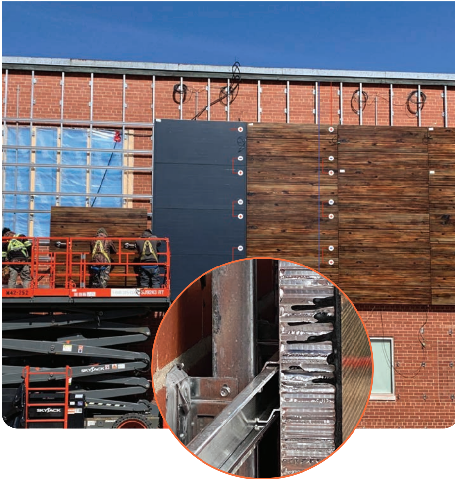
Interlocking Channels Attachment System.
