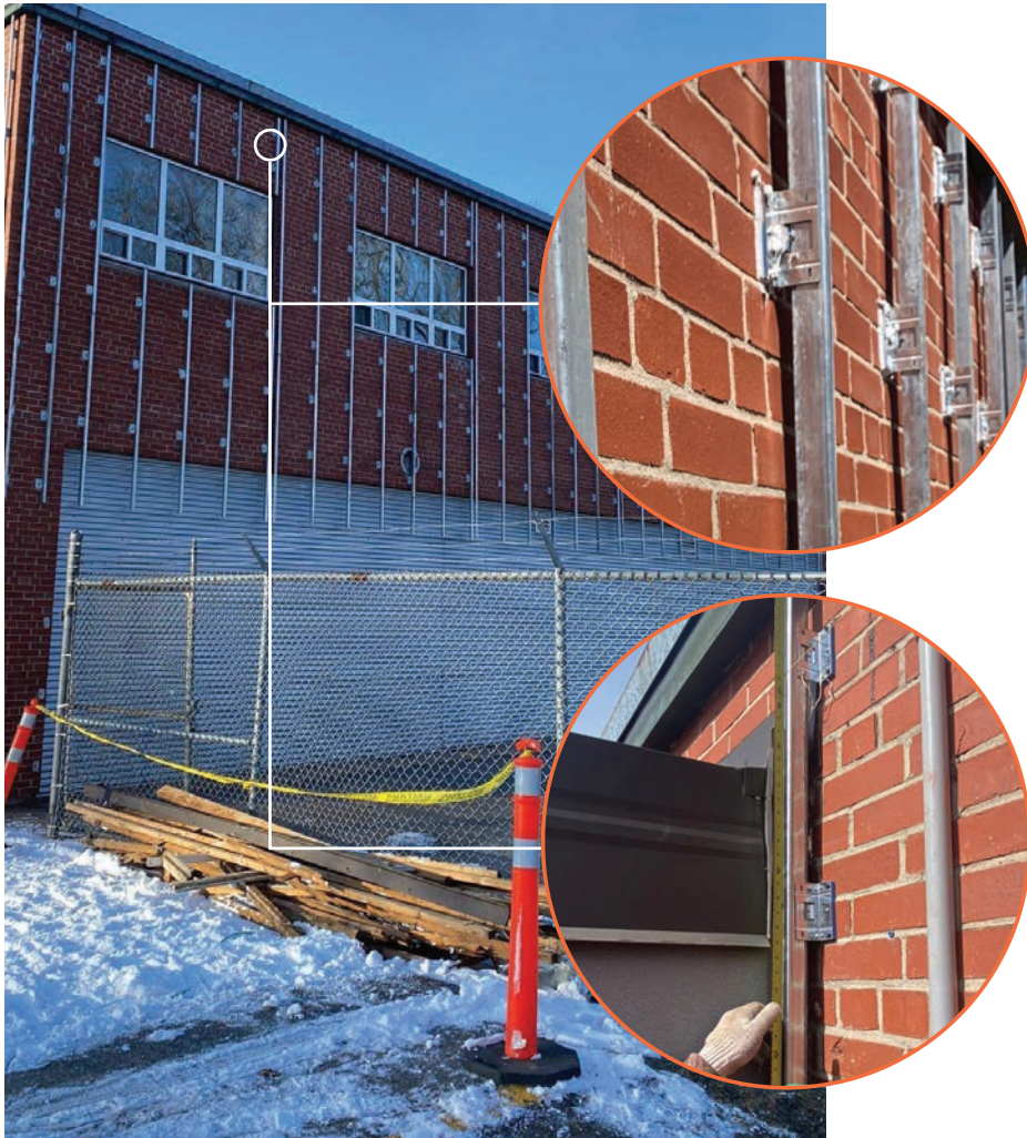
16 Gauge GS - 1.5" x 1.5" L-Angle
